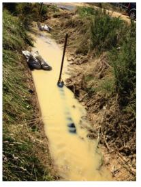
The picture above shows the passive application of HaloKlear DPS. That day, water was being diverted down the culvert from another location and the rain activated floc sheds wouldn't have operated.
